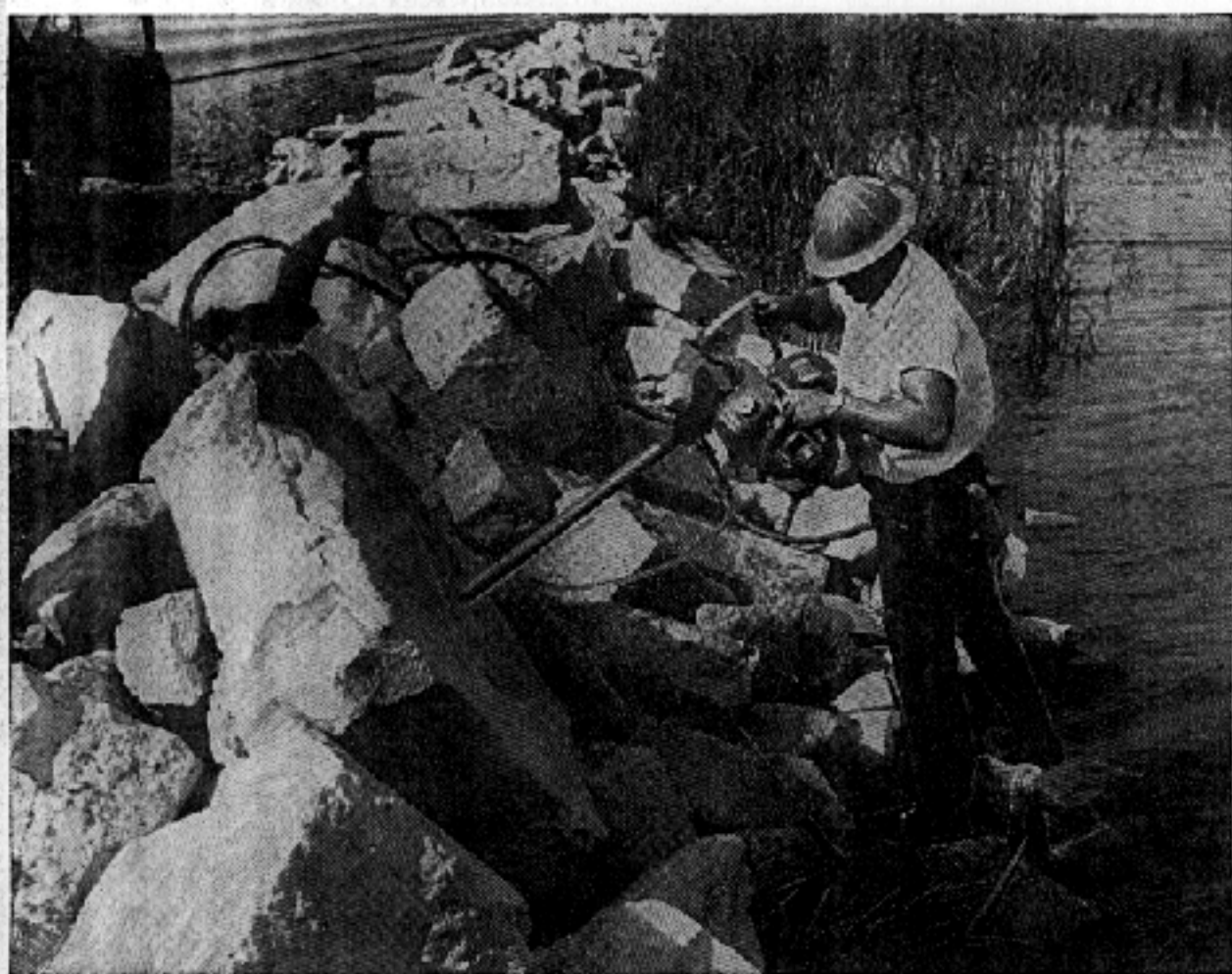
New portable coring tool replaces heavier, more expensive equipment, samples rock to depth of 50 feet
